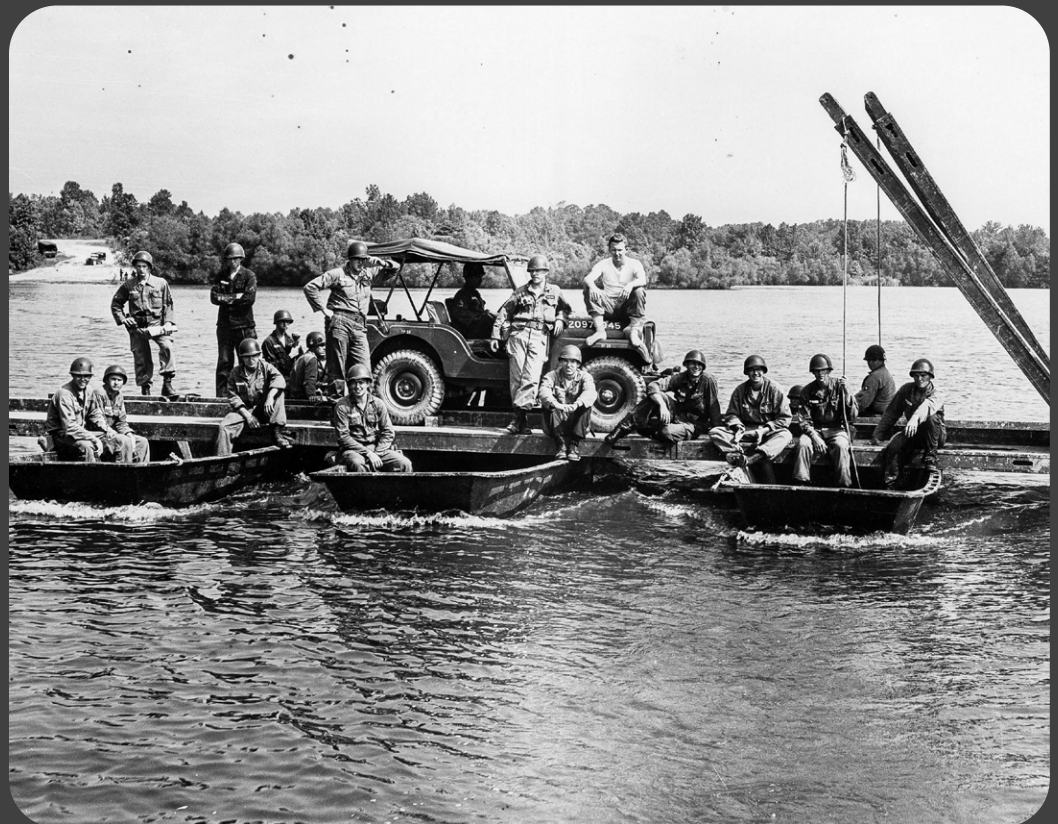
Soldiers from Company B, 112th Engineer Battalion test their "do it yourself" ferry on Des Islet Lake, Camp Breckinridge, Ky., 1958.
