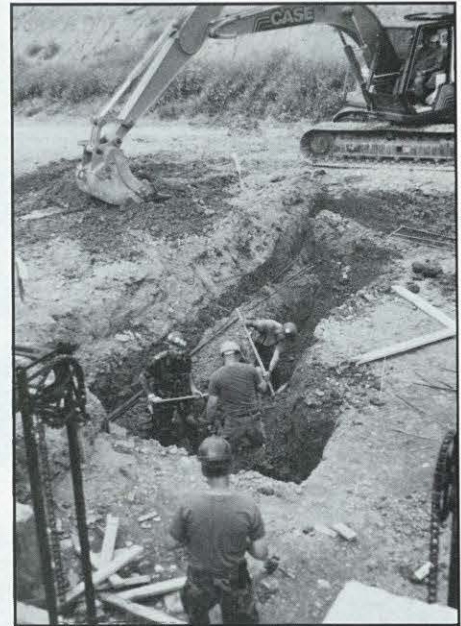
ABOVE: Members of the 200th Red Horse download pre-cast target shed walls from low-boy trailer. RIGHT: Personnel excavate target shed footings using power excavation equipment and hand digging operations.
