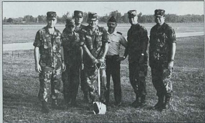
Col. James Caldwell and members of his staff break ground on the RETS rifle range. Caldwell has since been replaced by Col. Joseph C. Bowsher as commander of Camp Perry.
