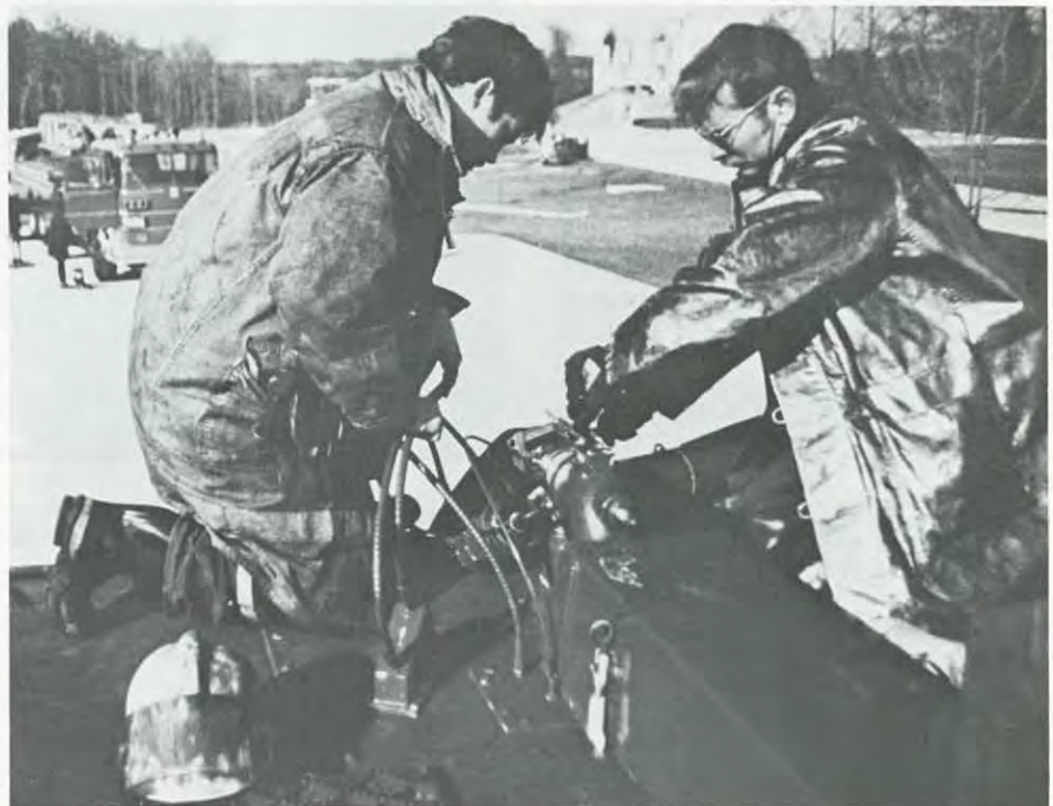
HOOKING IT UP — SRA Robert Mayberry and TSgt. Gary Studer install a special coupling device developed by the Toledo Fire Division and the 180th that allows a hook-up between Guard and civilian fire trucks.
