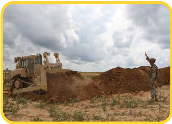
Sgt. Matthew Fuller, an equipment operator with the 1192nd Engineer Company, guides another operator during a berm emplacement for field artillery equipment during rotation 15-10 at the Joint Readiness Training Center, Camp Polk, La.
