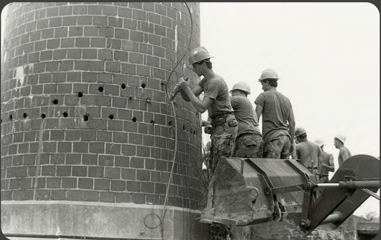
Soldiers from Company C, 112th Engineer Battalion place explosives charges on the outside of a chimney at Camp Atterbury, Ind., on June 21, 1991, prior to demolishing the structure.
