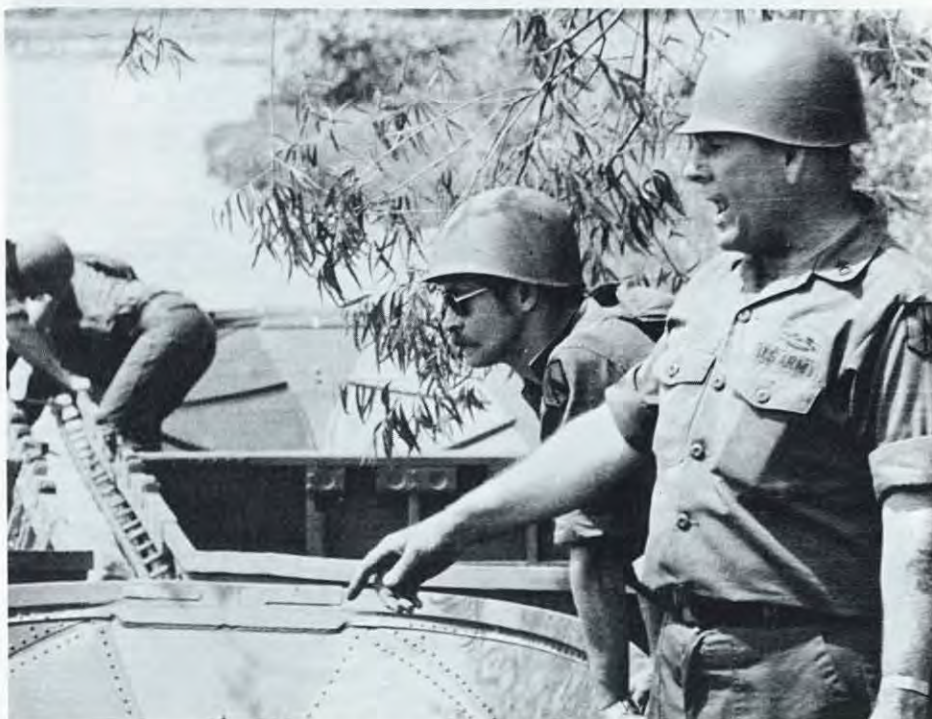
RAFT BUILDING —Platoon Sergeant Paul Binkley, of Lima, directs construction of a Light Tactical Raft during National Guard exercises at Fort Campbell. Completed in about 35 minutes, the raft is capable of floating a fully loaded 2½ ton truck and is used to transport initial personnel and equipment while primary bridges are being constructed. Shown also is Specialist Robert Reynolds of Ottawa, Ohio. (PHOTO BY SP4 RON TYLER).
