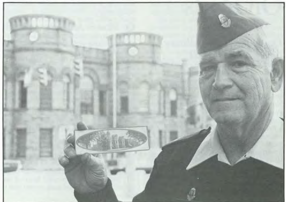
When the Kenton Armory was built in 1895, buggies and horses brought soldiers to drill. Although times have changed, the building remains virtually unchanged. Staff Sgt. Tracy Stanley, pictured here, has been serving the Ohio Army National Guard here for 20 years.
